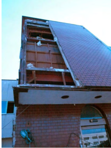
Drop of exterior wall of steel structure (Oroshimachi)
