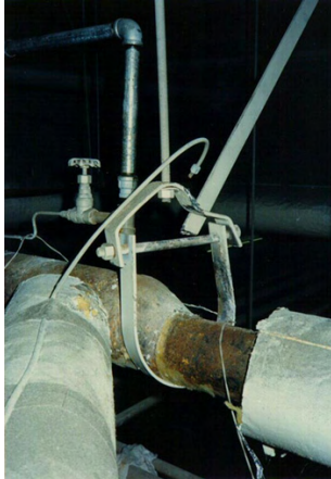
Pipe brace failed at connection in 1994 Northridge Earthquake
