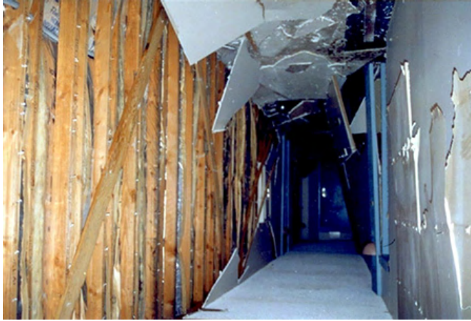
Damage to wood stud wall spanning floor-to-floor in the 1994 Northridge Earthquake
