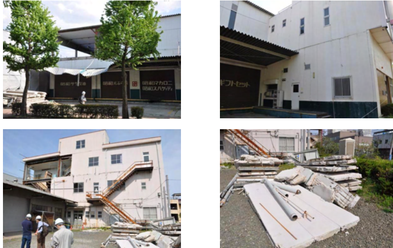
Exterior cladding damage, (Photos courtesy of Dr. Dimitrios Lignos)
