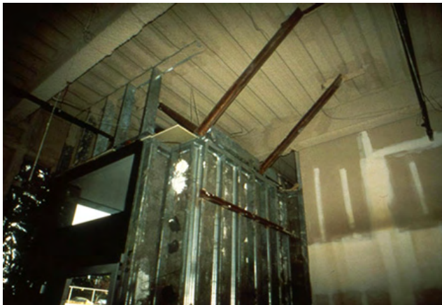
Out-of-plane bracing of partial-height metal stud partition to floor slab above
