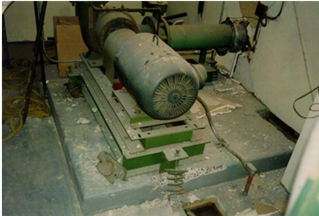
Failure of pump mounted on three vibration isolators including damage at wall penetration in the 1994 Northridge Earthquake
