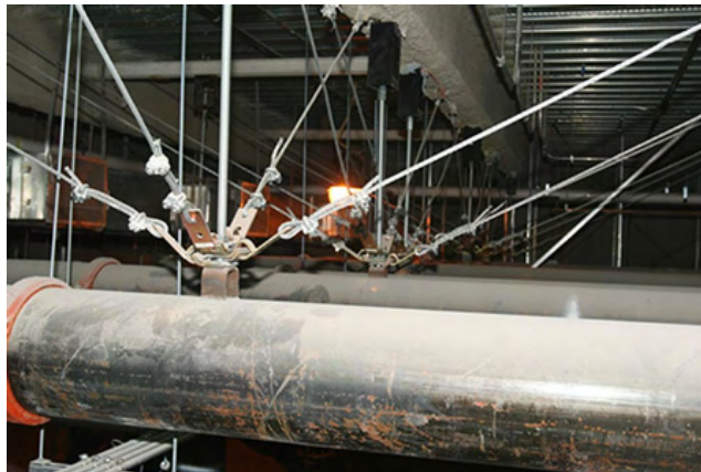
All-directional cable bracing of suspended piping; rod and cables attached to welded lug
