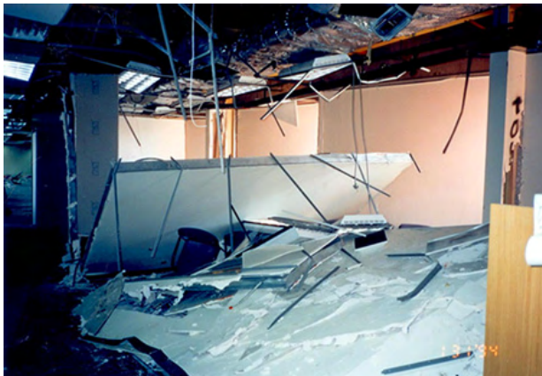
Failure of inadequately braced partial-height metal stud partitions in the 1994 Northridge Earthquake
