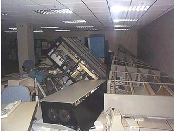
Damage to communication and computer racks
