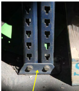
Well-anchored at the base
