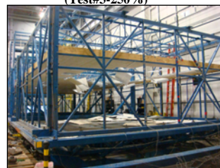
System Collapsed (Test#5-200%)
