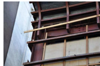
Exterior cladding damage. (Photos courtesy of Dr. Dimitrios Lignos)
