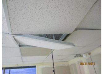
5 th floor ceiling failure
