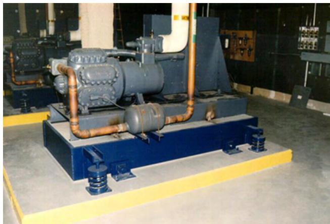
Open springs in conjunction with snubbers used to support equipment
