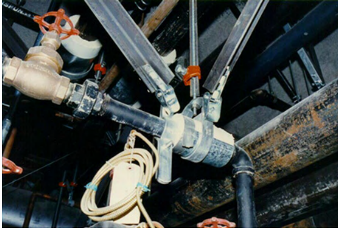
Pipe clamp used for longitudinal angle brace; note pipe clamp in direct contact with pipe. Clevis hanger used for transverse brace
