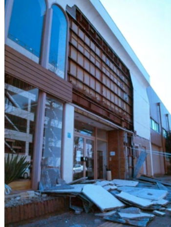
Drop of exterior wall of steel structure (Oroshimachi)
