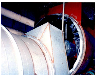
Sheet metal duct separated from suspended fan unit (Photo from FEMA E-74 courtesy of Wiss, Jenney, Elstner Associates)
