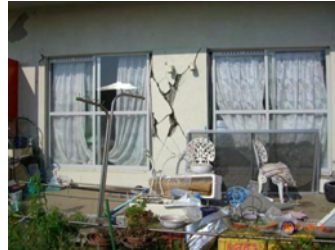
Shear cracks in non-structural components, (Photo courtesy of Dr. Dimitrios Lignos)
