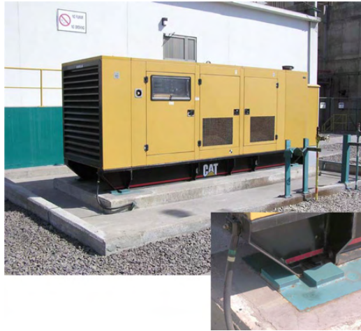
Emergency generator with skid mount on housekeeping pad; shear lugs added following the 2001 Peru Earthquake
