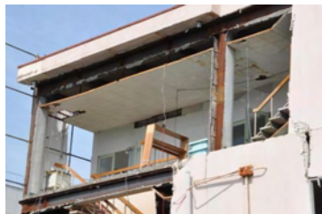
Moment frame: no damage
