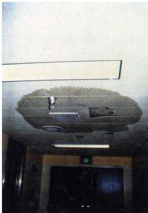
Leakage caused by pipe damage at joint; 1994 M6.7 Northridge Earthquake
