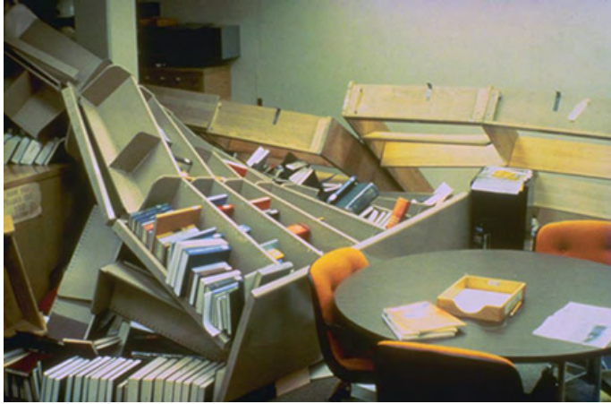
Failure of poorly anchored wood and metal book shelves at the Lawrence Livermore Laboratory, Livermore, California
