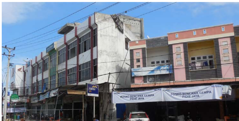
Figure 7. Typical shop-house in the affected area (photo: Muhammad Riyansyah).
