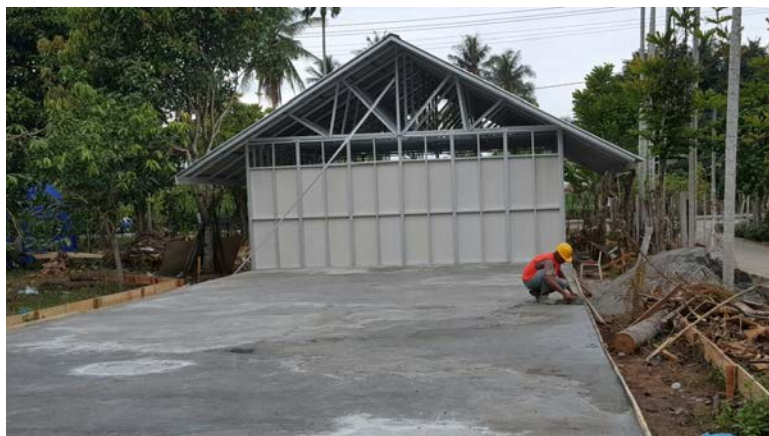
Figure 26. Construction of temporary school (photo: Puskim Kemenpupera). 12
