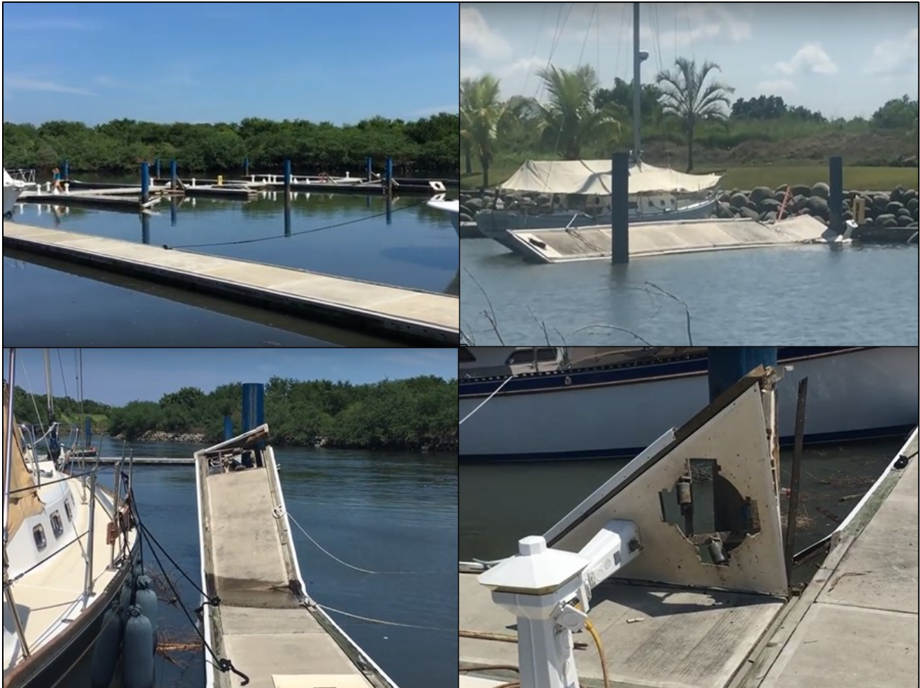
Figure 4 Video screen captures of dock damage in Marina Chiapas the day after the September 7, 2017, earthquake. According to the videographer, the amplitude of the tsunami in this area was several meters causing the floating docks to overtop the piles, and damage to the docks themselves (video link: https://www.youtube.com/watch?v=bBBVt1wLM9g ).
