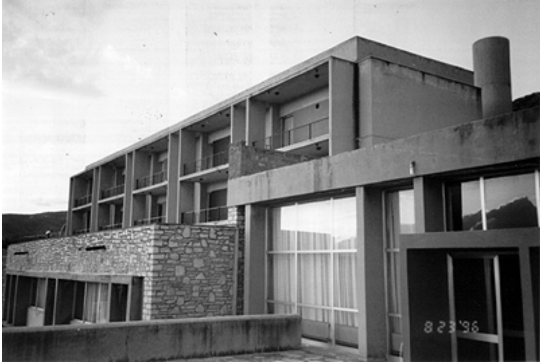
Fig. 19 Undamaged R/C building (GREEN)
