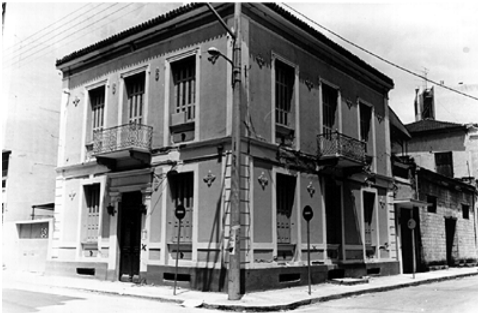
Fig. 6 Practically undamaged, 2-storey masonry building (GREEN)
