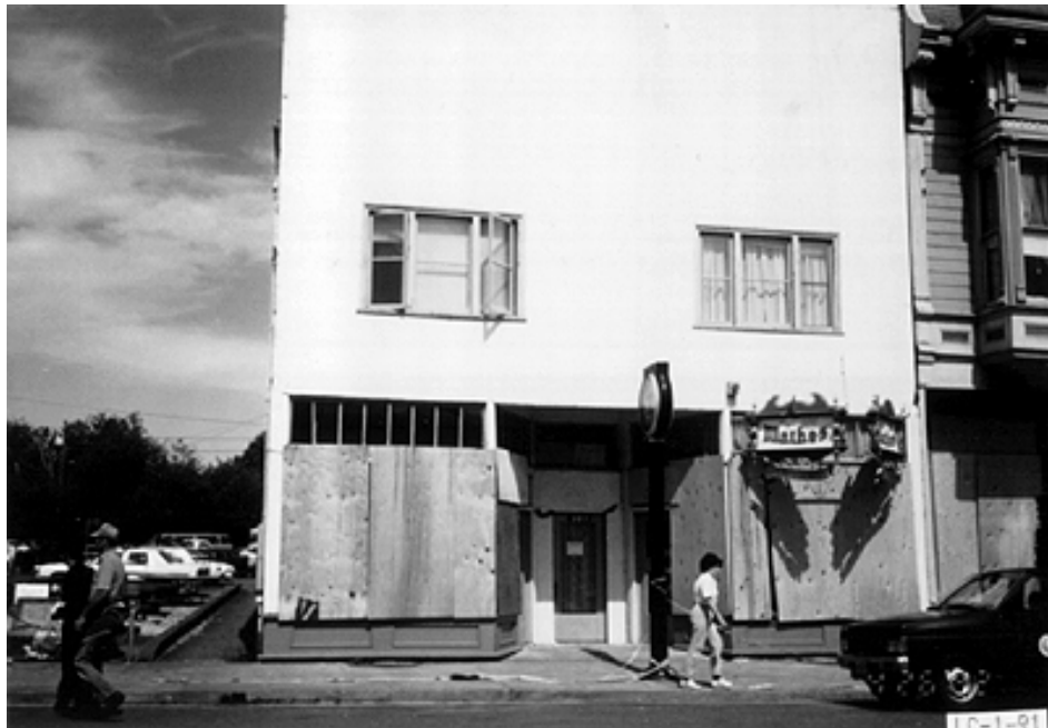
Fig. 13 Damaged 2-storey wood frame building. Lots of broken glass and some lateral offset (YELLOW)
