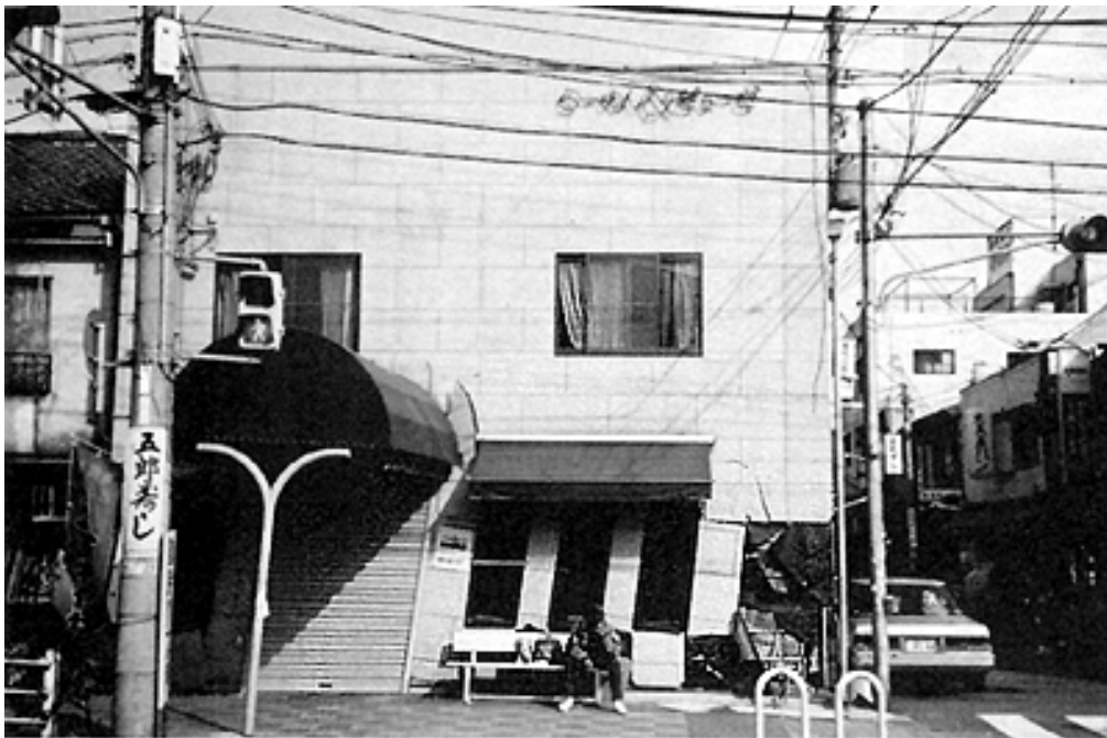
Fig. 18 Large racking of 2-story wood frame building (RED)
