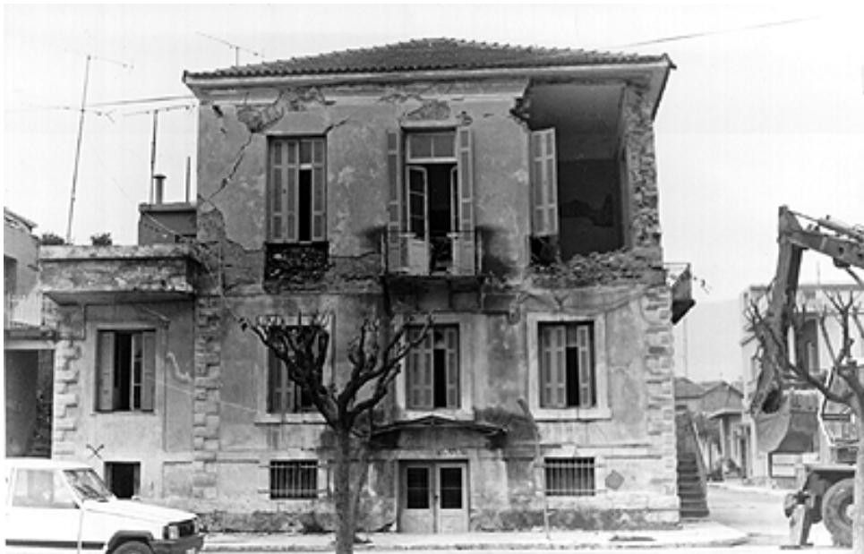
Fig. 12 Partial collapse of masonry building (RED)
