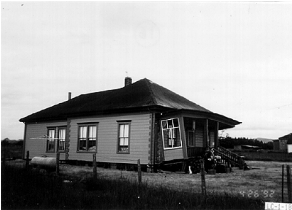
Fig. 16 Single story wood frame house slipped off its foundation (RED)
