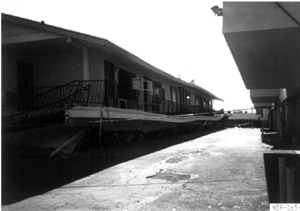
Fig. 17 Collapsed 2-story wood frame apartment building (RED)
