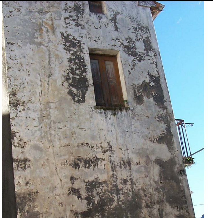
Fig. 4.2: Vertical cracks in the spandrel beam between the two openings (type 1) and along the left transversal wall (type 6).
