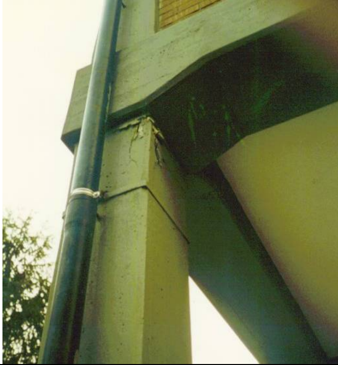
Fig. 4.28 Concrete spalling at the column top section, slight vertical cracks. Damage grade: D2-D3 (Bagnolo, RE, 1996)
