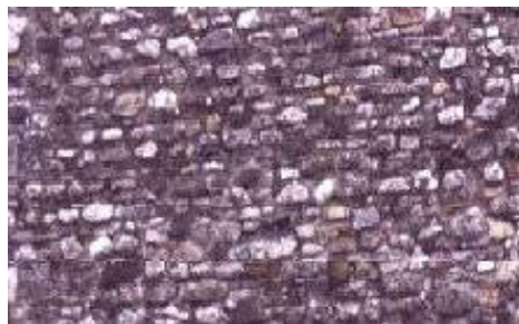
Benevento: rubble stone with fairly regular layout
