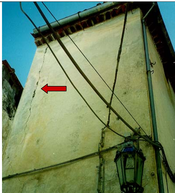
Fig. 4.10 Vertical crack with separation of the orthogonal walls (type 7). Damage grade: D2-D3
