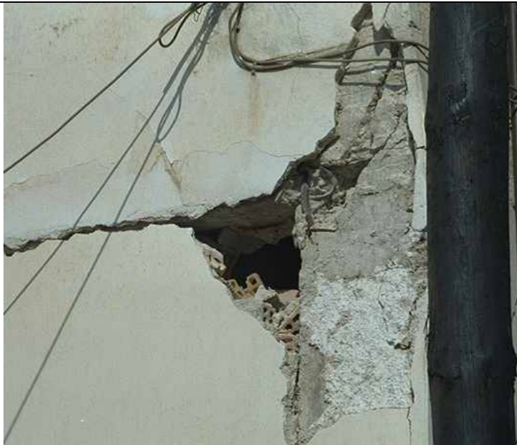
Fig. 4.29 Damage to the beam- column joint with concrete spalling. Crushing of the infill panel. Damage level to vertical structures: D4
