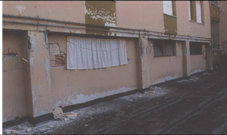
Fig. 4.27 Cracks in several columns, facilitated by oxidation of the reinforcement. Insufficient stirrups. Total damage grade to vertical structures: D2- D3 (Fabriano, 1997)
